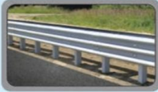
Thrie Beam Guardrail
