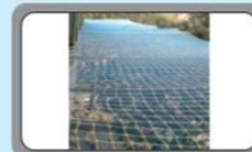
Under Construction Safety net
