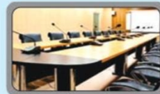
Conference Room PA System
