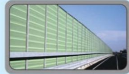
Sound Proofing Barrier
